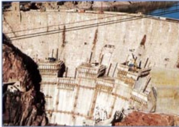
Roosevelt Dam, Arizona
